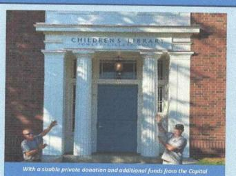
Renovation Campaign, a total refresh of the Children's Library entry with new window glazing, paint, copper flashing and wrought iron handrail, maintoining the historical integrity of the Fowler Gillette house and stabilizing the entrance structure for the future.
